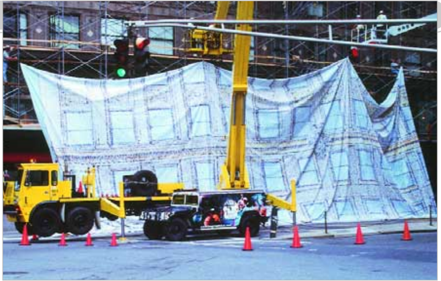
The material used was Ultra Mesh from Ultra Flex. It took about 65 hours to print, and when assembled, the graphic measured 110' X 128' and weighed 1,400 lbs.
